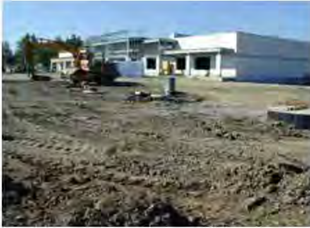
Figure 22.2. Construction activities cause bare compacted soil with potential for water and wind erosion, and challenges with revegetation.
