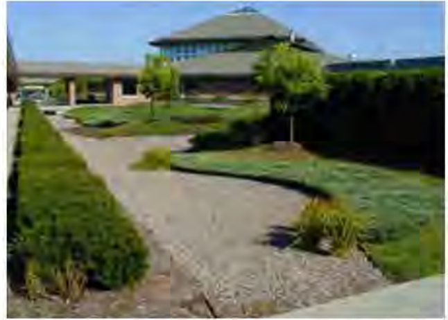
Figure 22.8. Retention of urban stormwater. Left: A swale that contains runoff from a parking lot in the distance. Right: Gravel-based swale with subsurface drains (under gravel) that captures roof runoff from a regional airport terminal.
