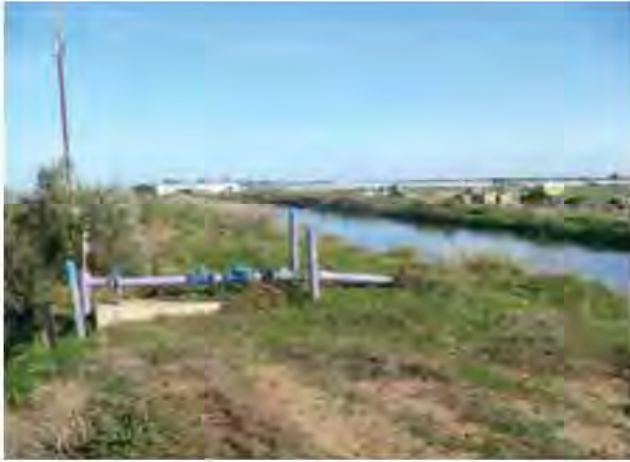
Figure 17.5. Recycled wastewater from the City of Adelaide, Australia, is pumped into an irrigation pond for a vegetable farm. Wastewater-conveying pipes are painted purple to distinguish them from freshwater conduits.
