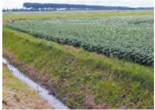
Figure 17.13. Left: the Wouda pumping station was built to drain large areas in Friesland, Netherlands, and is the largest steam pumping station ever built. It is now on the World Heritage List. Right: A drainage ditch removes excess water and lowers the water table in newly developed lands ("polders") in the Netherlands.
