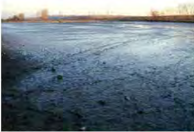
Figure 14.10. Top: A sediment control basin in a Central European landscape where conventional tillage is widely used. Bottom: Sediment regularly fills the basin and needs to be dredged.
