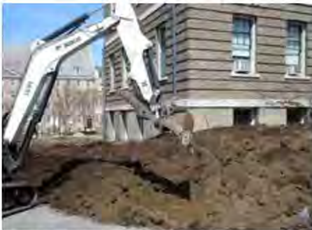
Figure 22.5. Left: scoop-and-dump method for de-compaction of soil and mixing in compost. Right: Ameliorated soil with plantings and mulch. Photos by Cornell University, Urban Horticulture Institute.
